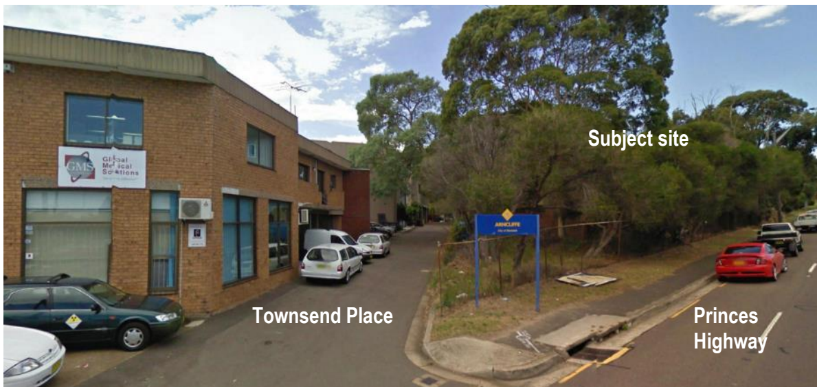
Character of Townsend Place which forms the south western boundary of the site
